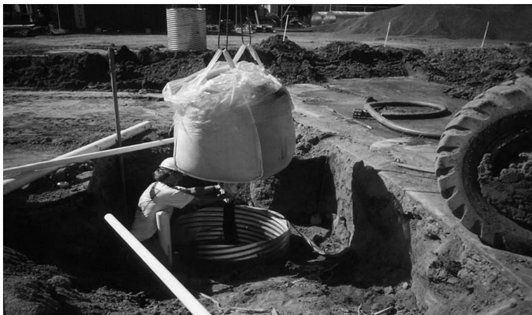
FIGURE 14.5 Filling gate tank with granular activated carbon.
