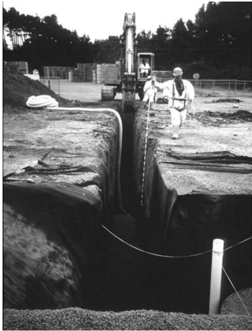
FIGURE 14.6 Collector line installation for funnel and gate system.
