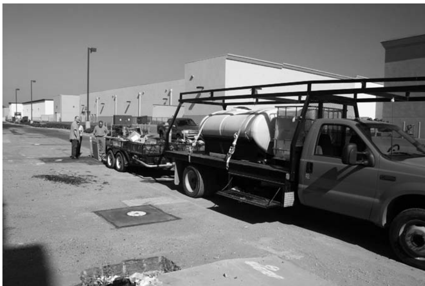
FIGURE 13.35 Reagent injection setup. Concentrated reagent solution is carried in a stock tank on the truck bed. Dilution water is drawn from a nearby hydrant and reagent mixing and pumping occurs on the attached trailer.
