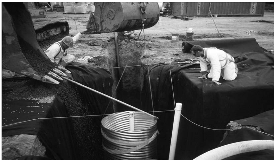
FIGURE 14.4 Funnel and gate system, showing final connection of collector lines to gate tank.
