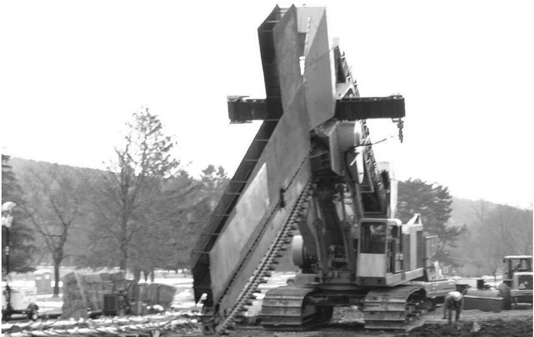
FIGURE 14.9 One-pass trencher preparing to install permeable zero-valent iron reactive wall.
