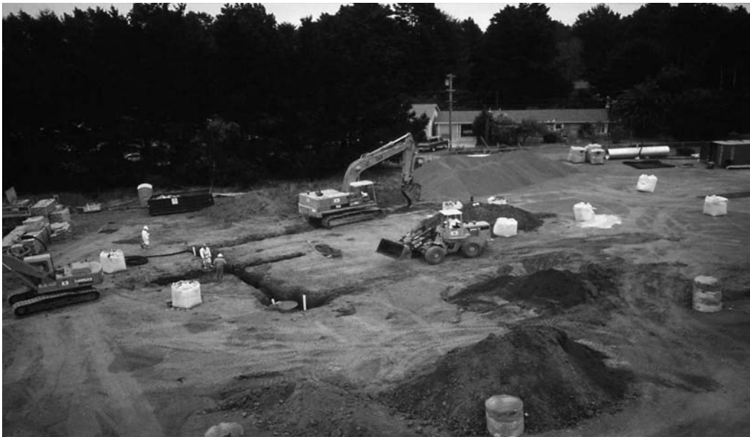
FIGURE 14.2 Overhead view of funnel and gate system construction.
