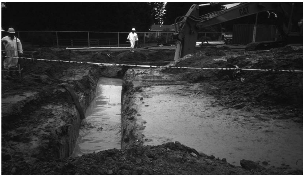
FIGURE 14.7 Constructing the slurry wall component of a funnel and gate system.
