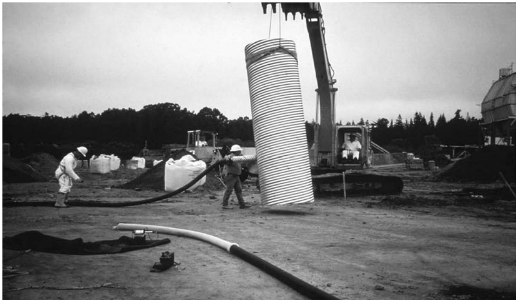
FIGURE 14.3 Funnel and gate construction, showing setup of activated carbon gate.
