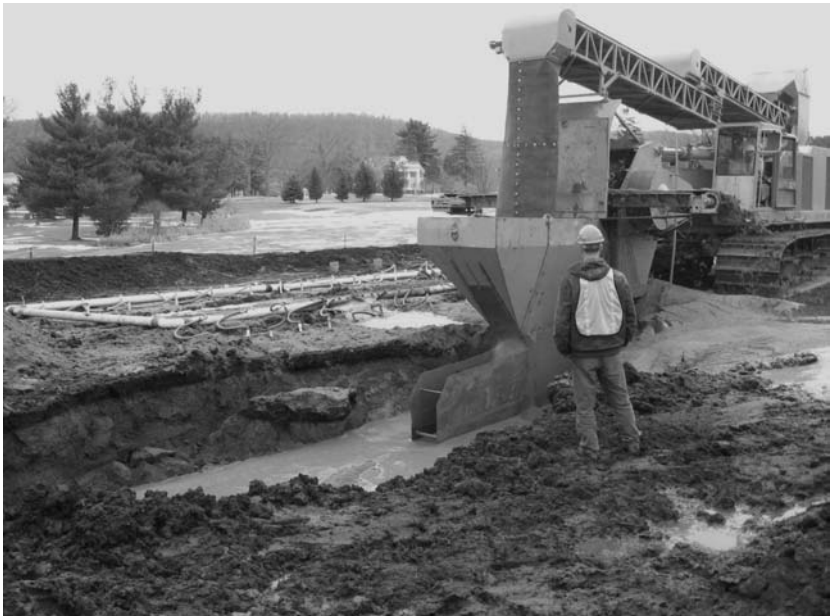
FIGURE 14.10 One-pass trencher installing zero-valent iron and sand slurry to a 35-foot depth.
