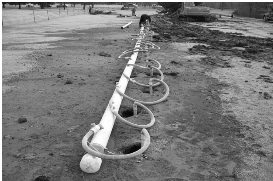
FIGURE 14.8 Vacuum well point dewatering for groundwater suppression, prior to zero-valent iron reactive wall construction.
